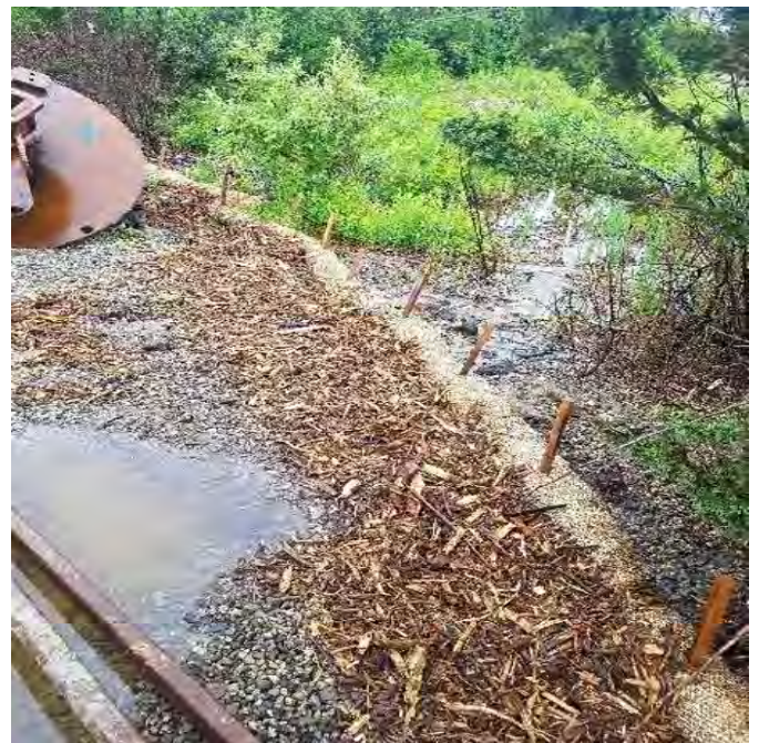
Fig 4: Combined berm installed around lay down yard cont. Viewing south. (6-11-19).
