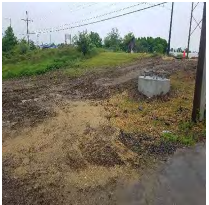
Fig 12: Foundation for Str. F107-136. A utility crew working along Woodbury Ave has excavated through the area that our crew finished and mulched with straw. There is now exposed soil in that area. (6-11-19).
