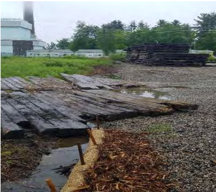
Fig 7: Combined berm installed around the lay down yard cont. Viewing north. (6-11-19).
