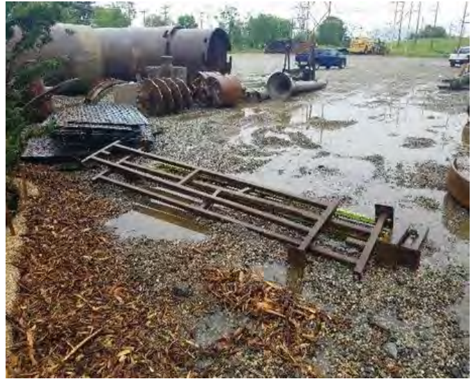
Fig 6: Combined berm installed around the lay down yard cont. Viewing northeast. (6-11-19).
