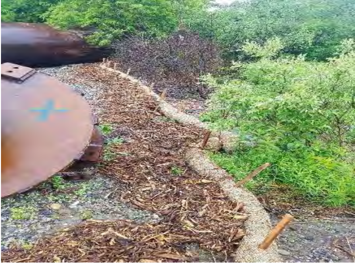
Fig 5: Combined berm installed around lay down yard cont. Viewing south. (6-11-19).
